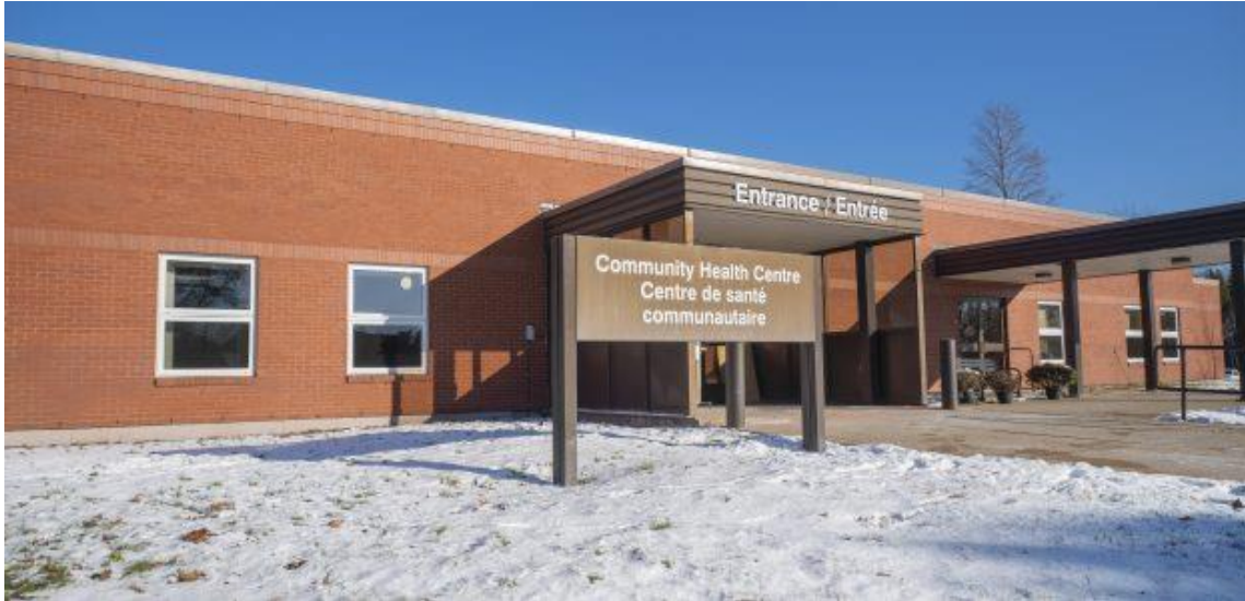
Figure 4-14 Queen's North Community Health Center in North Minto (Horizon Health Network, 2026)
