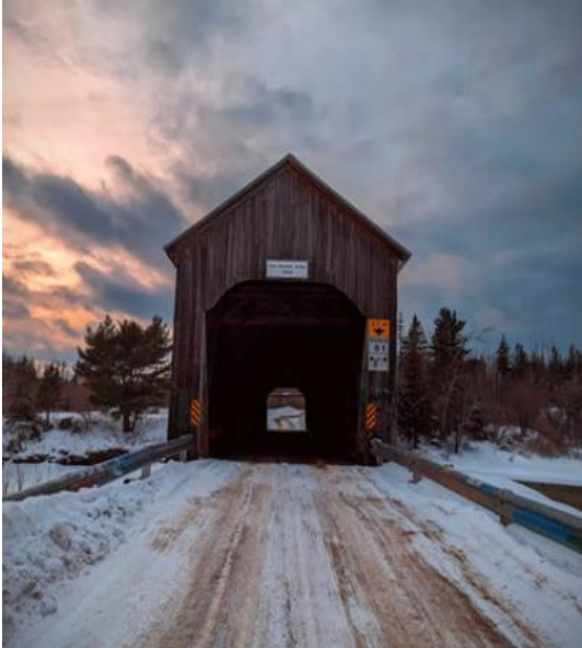
Burpee Bridge- Gaspereau
